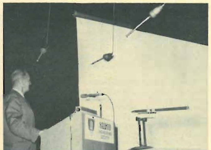
Overhead mikes pick up talker's voice even if he turns to side. Mike at lower right is used for questions from audience.
